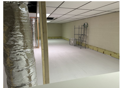
Second floor collections storage area.
